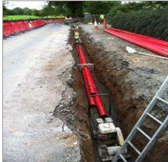
Figure 2 - Typical 110kV Underground Duct Installation
