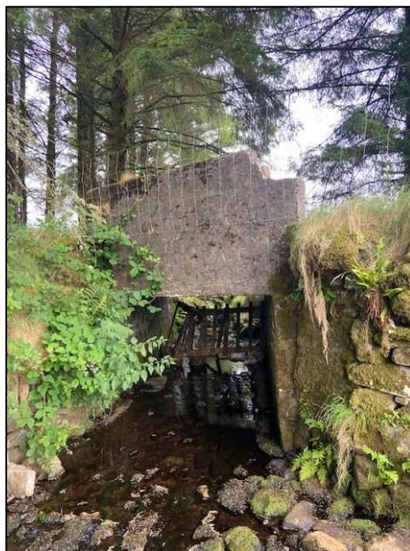
Figure 14 - Bridge 1 within L-74001-1
