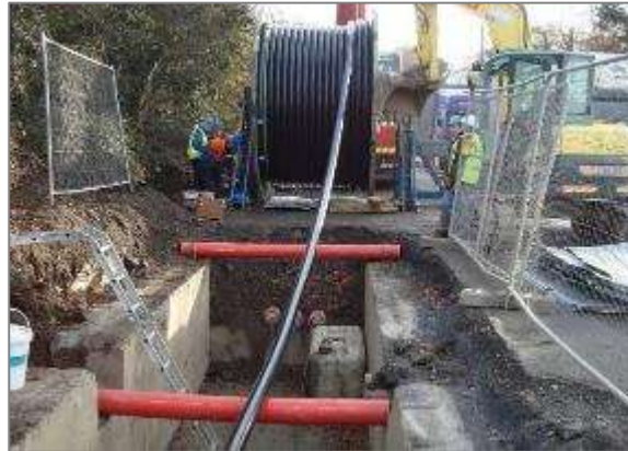
Figure 10 - HV cable pulling procedure (Typical drum set-up)
