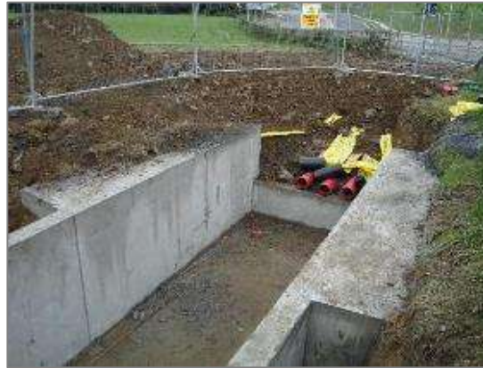
Figure 8 - Completed joint bay prior to cable installation (in-situ)
