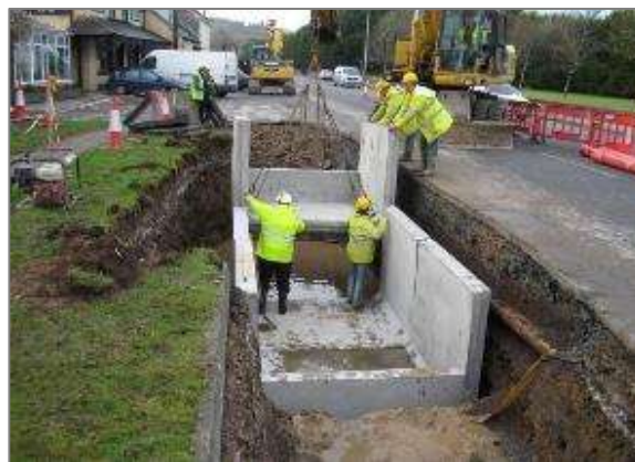
Figure 9 - Typical joint bay under construction (pre-cast)
