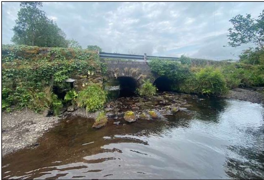
Figure 18 - Droichead Uí Mhathúna crossing the Sullane River along the L-3400-32 roadway
