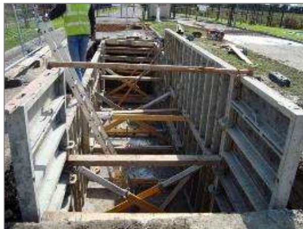
Figure 7- Typical joint bay under construction (in-situ)
